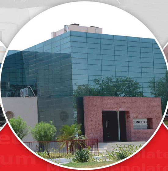
API Facility Dholka, Ahmedabad, India
